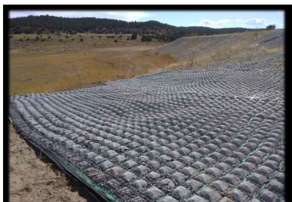
Figure 7: flexible concrete matting used for slope stabilization adjacent to the south shore.
