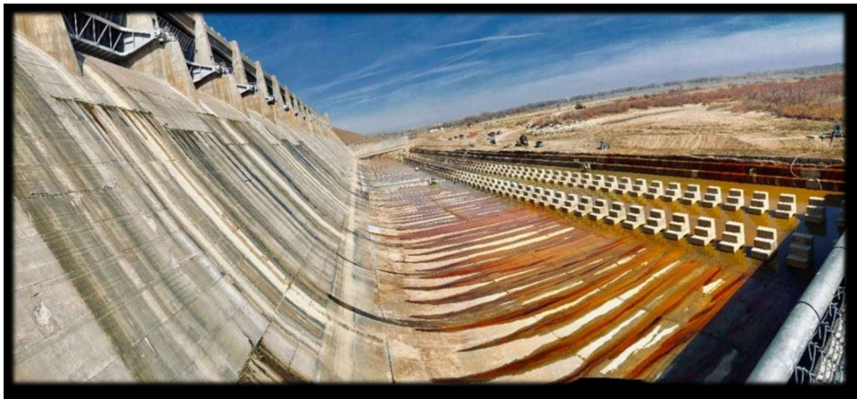
Figure 8: Stilling basin emptied, all sediment removed, and drain holes functioning properly.
