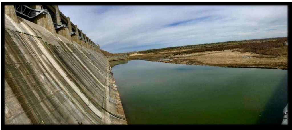
Figure 9: Stilling basin being filled.
