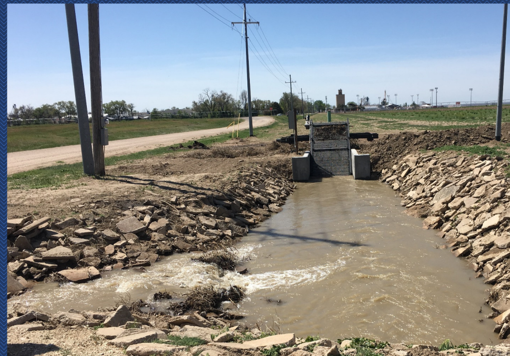
After: One Pipe
