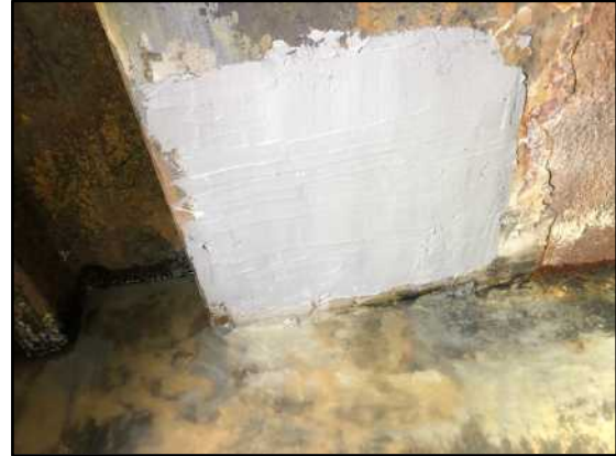
Figure 6: Metal repair patch in conduit liner
