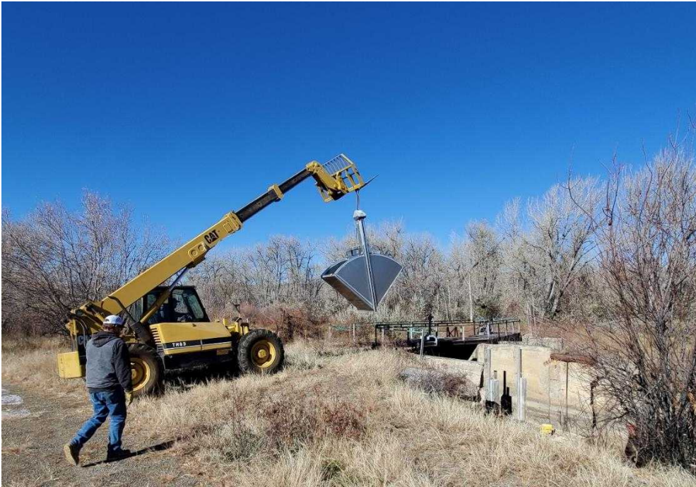
Enlarged Southside Ditch – New headgate installation – November 16, 2022
