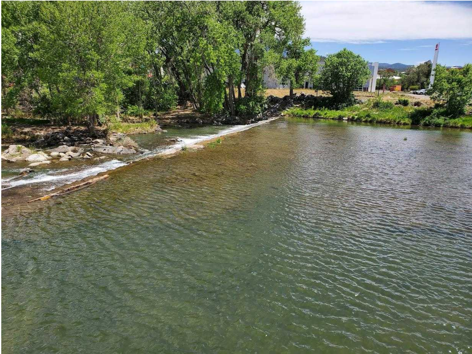
Baca/Picketwire Ditch Diversion Dam area with “Island” removed (March 2022).
