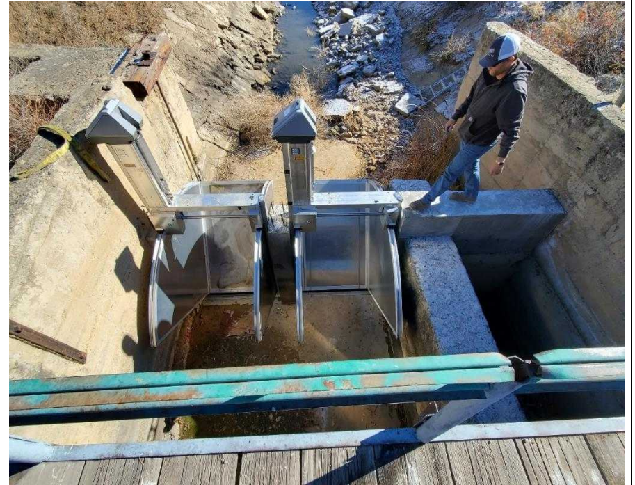
Enlarged Southside Ditch – New headgate installation – November 16, 2022
