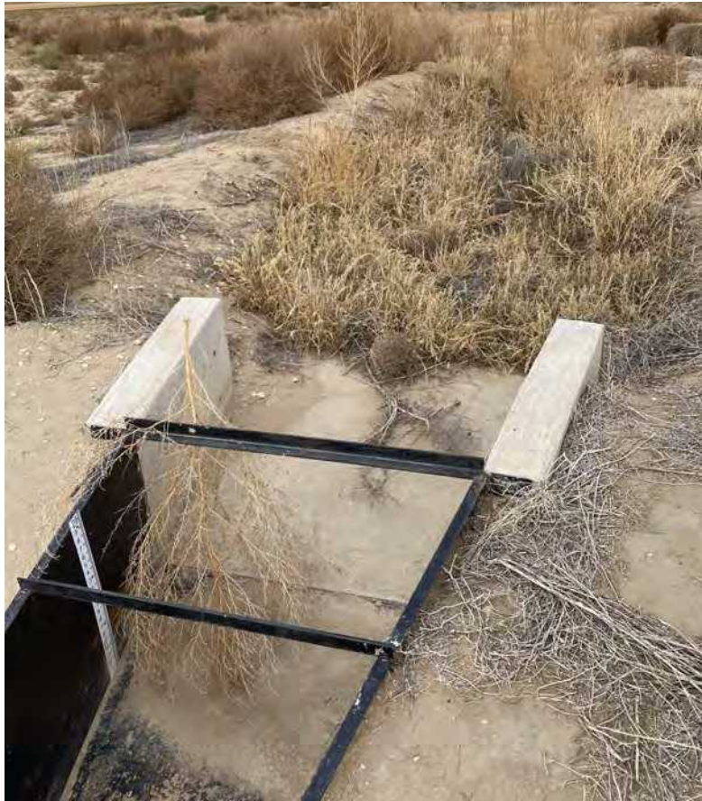
Figure A5 ARF27LCO Flume Upstream Mouth
