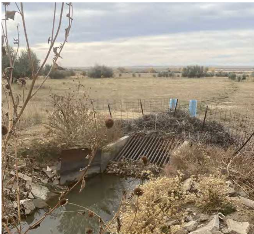
Figure A10 Horsecreek Augmentation Station Trash Rack
