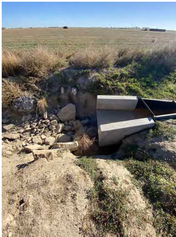
Figure A37 Farm 110 Storage Facility Outlet Flume Downstream Outlet
