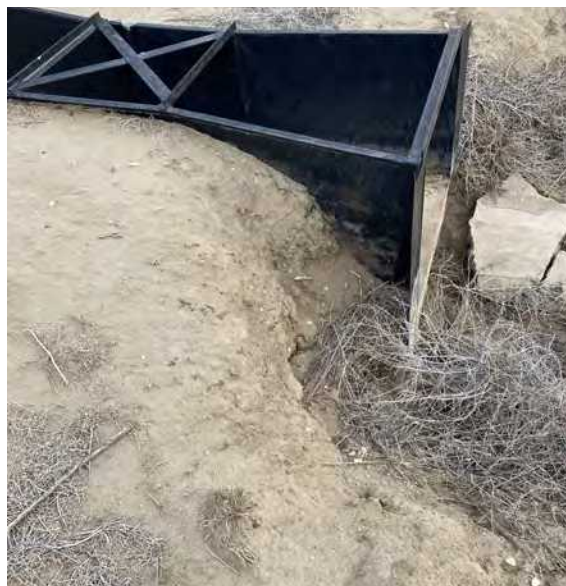
Figure A6 Farm 60 Recharge Facility Outlet Flume Downstream outlet
