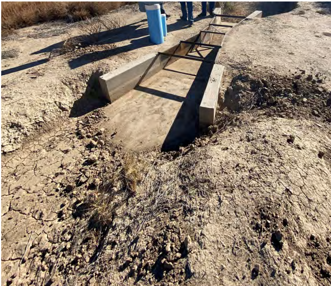
Figure A34 Farm 110 Recharge Outlet Flume Upstream stilling pool
