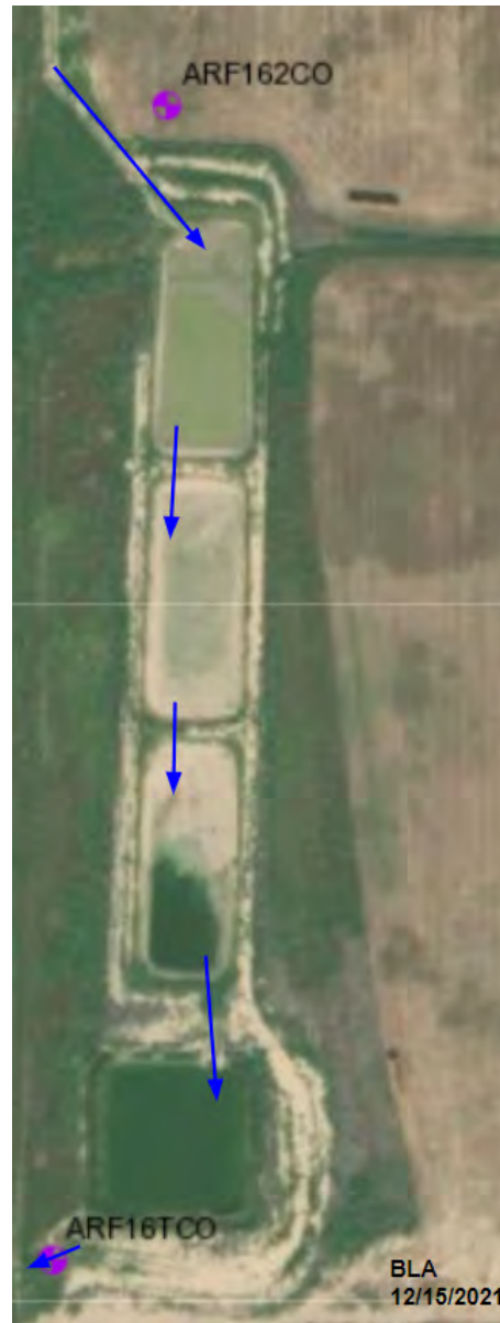
Figure A19 Farm 65 Recharge Facility Overview
