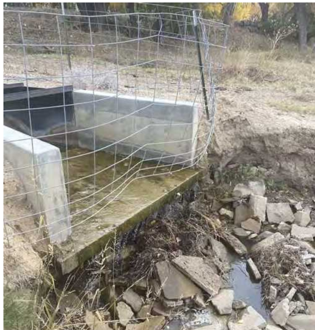
Figure A9 Horsecreek Augmentation Station Downstream Flume Exit
