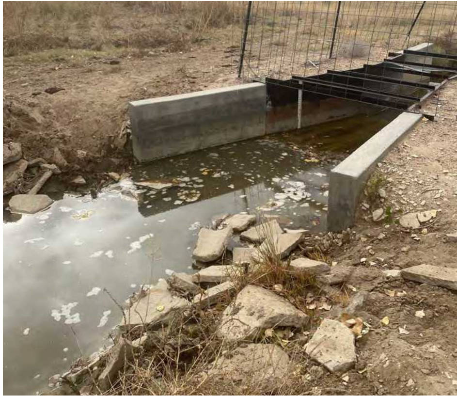
Figure A8 Horsecreek Augmentation Station Upstream Mouth Looking Downstream
