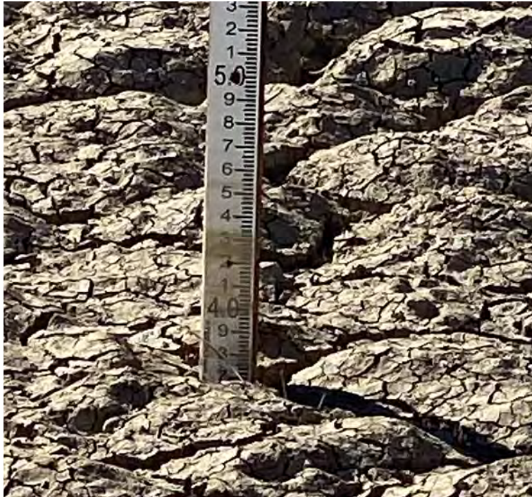
Figure A31 Farm 110 Recharge Facility Sediment Pond Staff Gage
