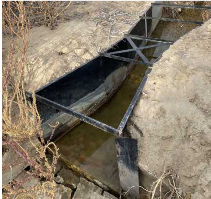
Figure A4 ARF027CO flume profile with waterline (facing upstream)
