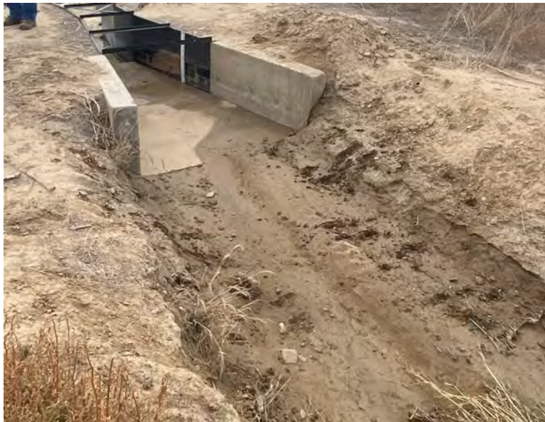
Figure A16 Farm 132/133 Inlet Flume (ARF14SCO) Upstream stilling pool
