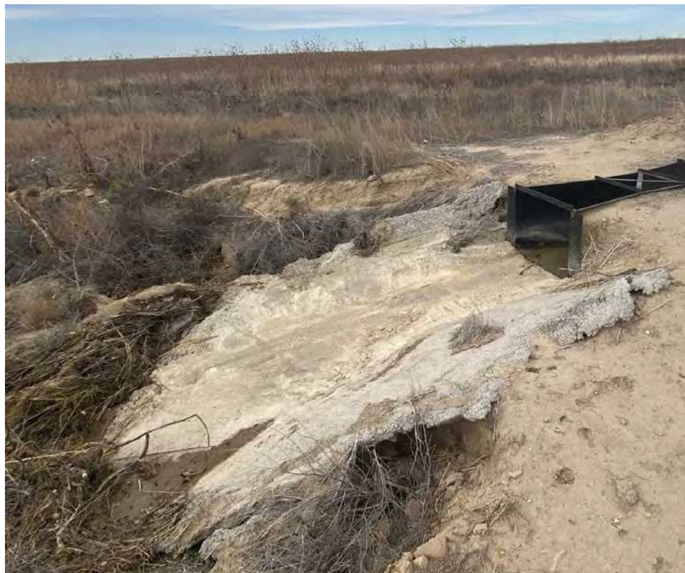
Figure A15 Farm 132/133 Inlet Flume (ARF14SCO) Downstream outlet
