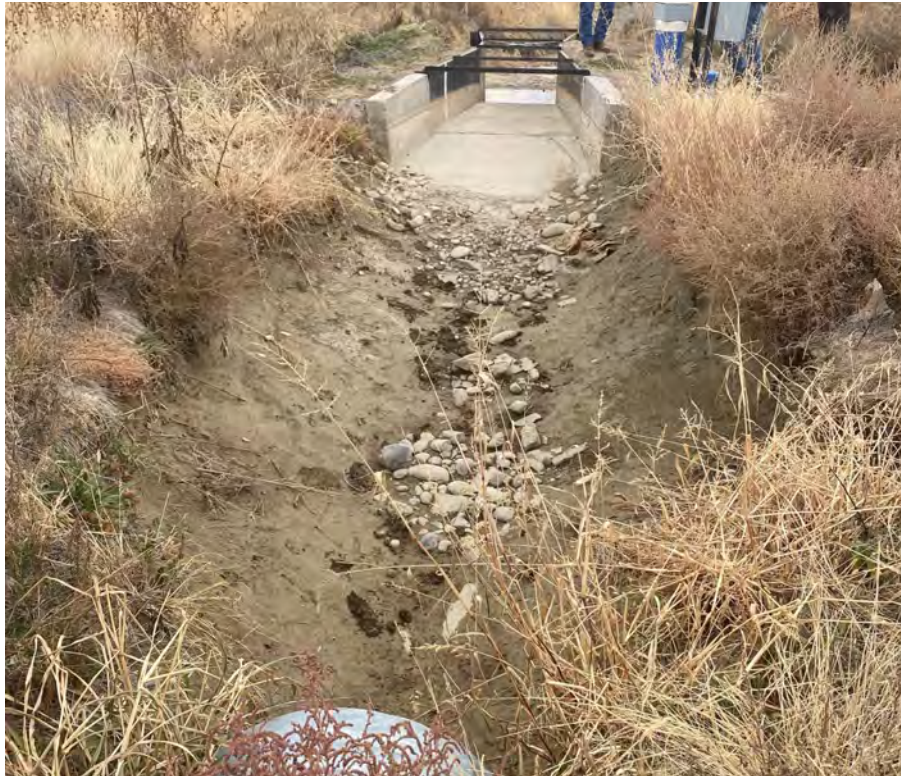
Figure A12 Lower Gageby Creek Augmentation Station Upstream Conditions
