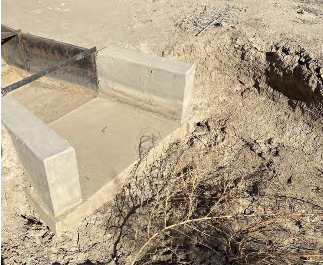
Figure A33 Farm 110 Recharge Outlet Flume Downstream outlet
