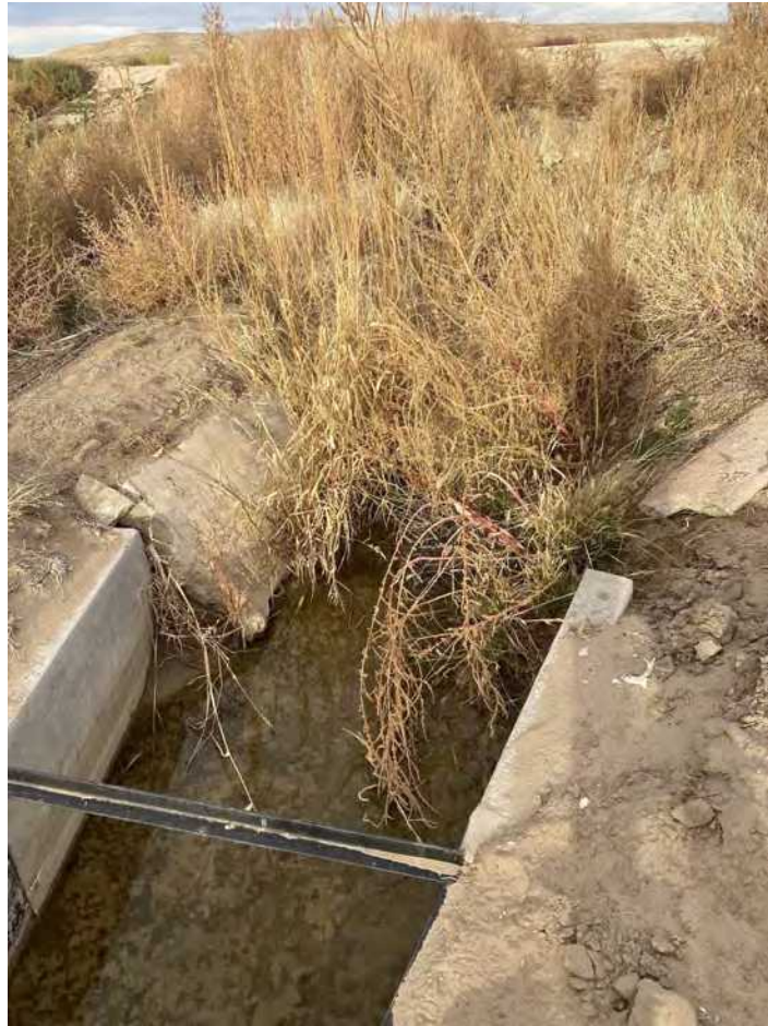
Figure A2 ARF027CO Flume Upstream Mouth
