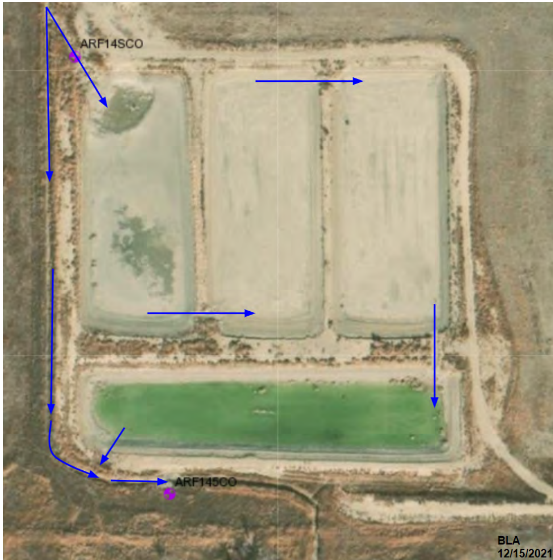
Figure A14 Farm 132/133 Recharge Facility Overview
