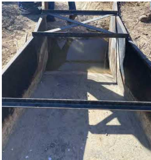
Figure A24 Wheatridge Augmentation Station Flume with waterlines indicating submergence.
