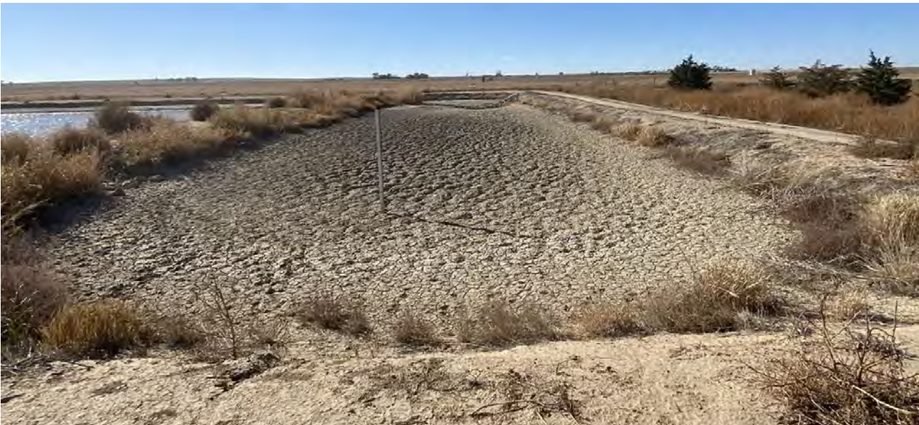
Figure A30 Farm 110 Recharge Facility Sediment Pond
