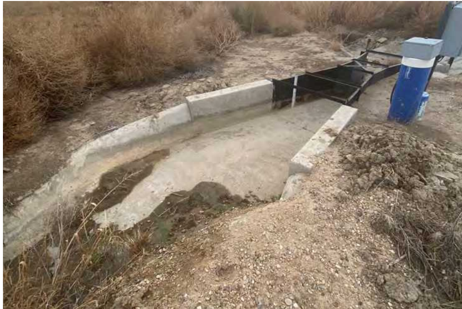
Figure A11 Upper Gageby Creek Augmentation Station upstream of flume, stilling pool
