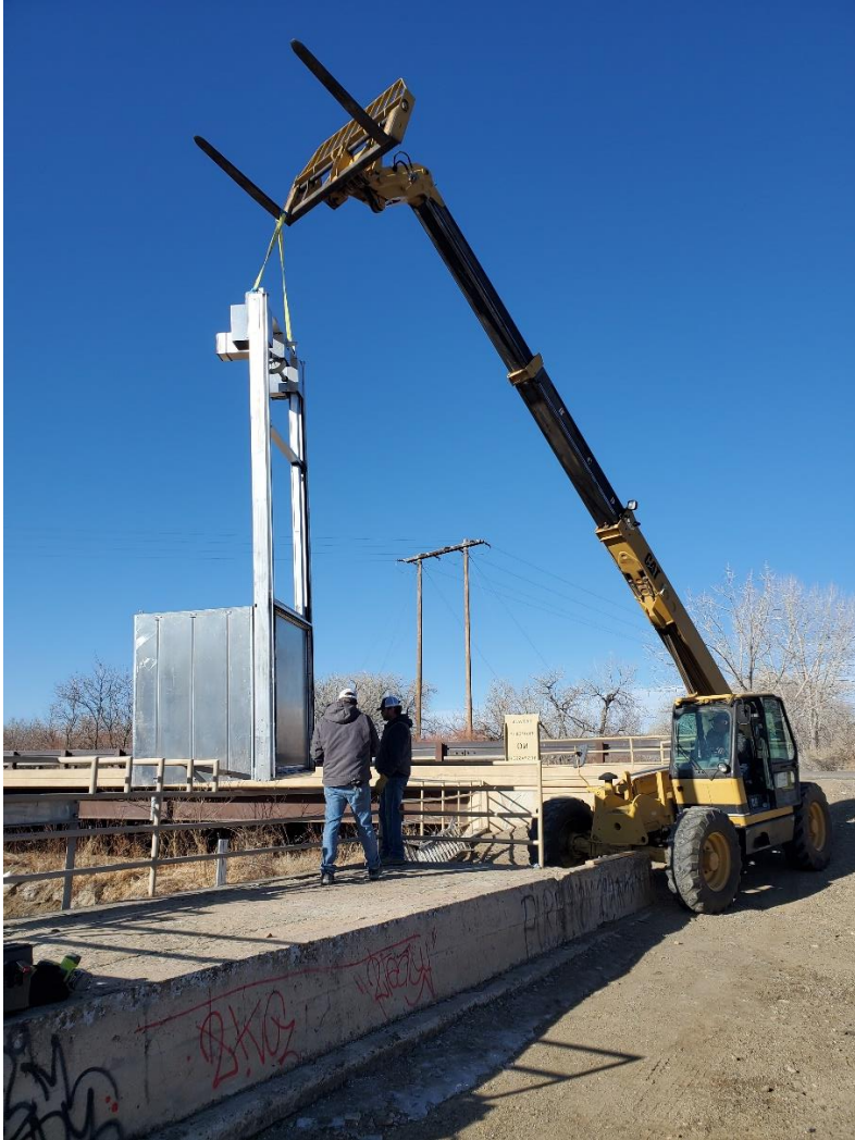
Model Canal – New headgate installation – March 2023
