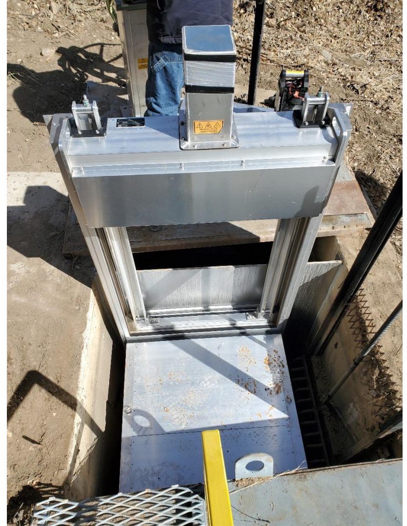
Hoehne Ditch – New headgate installation – March 2023
