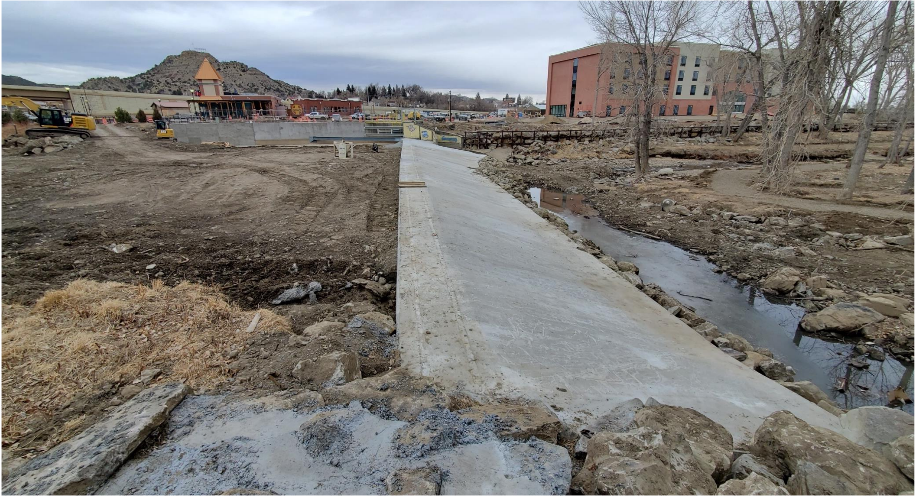
Picketwire/Baca Ditch Diversion Dam area with Dam Reconstructed (March 2023).
