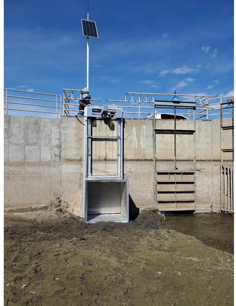
Model Canal – New headgate installation – March 2023
