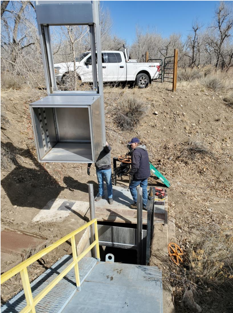
Hoehne Ditch – New headgate installation – March 2023
