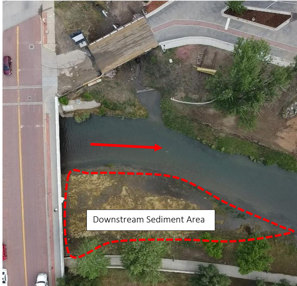
Commercial Street Bridge Area Sediment Removal (May 2023).
