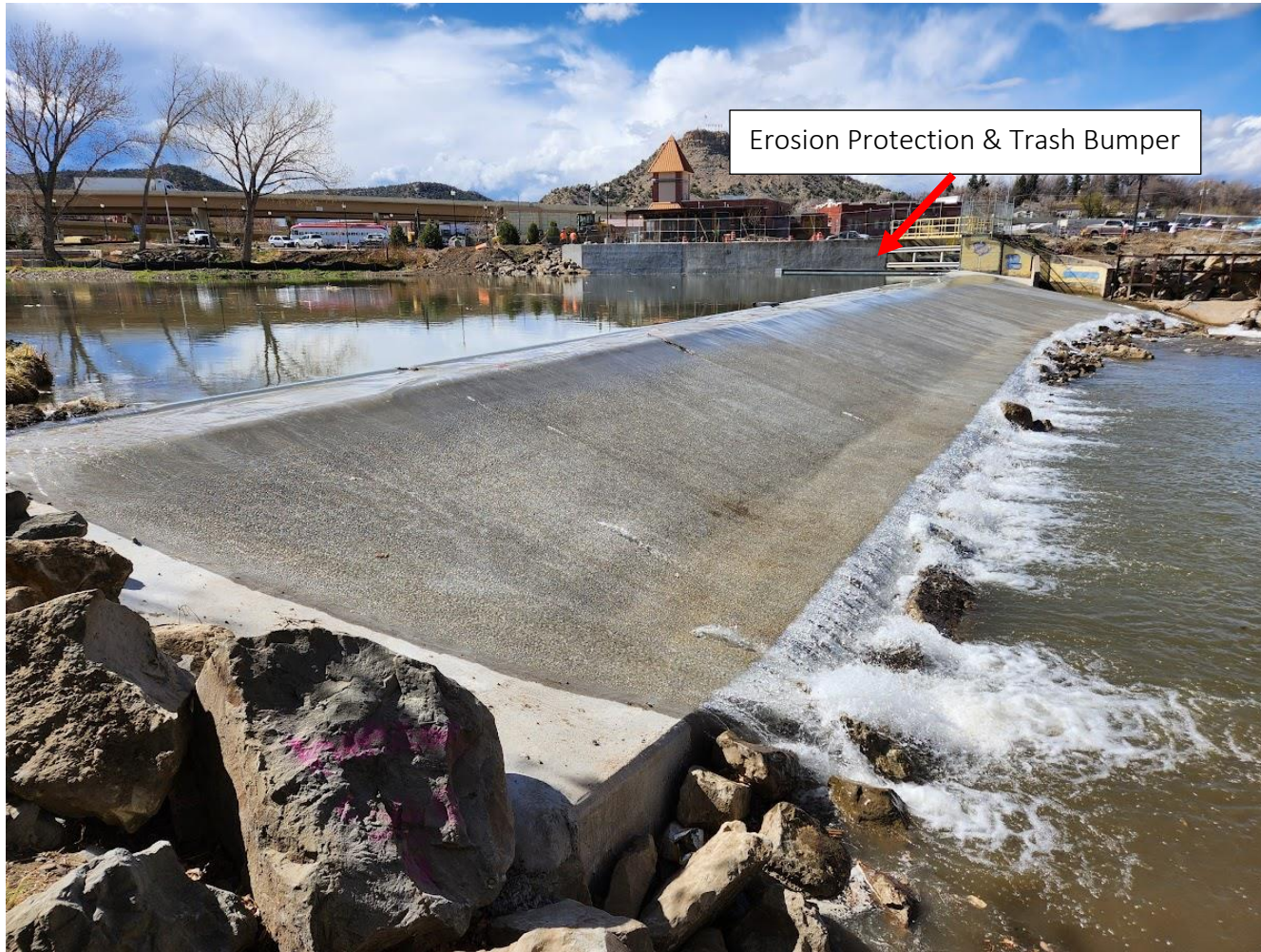
Picketwire/Baca Ditch Diversion Dam area with Dam Reconstructed (April 2023).
